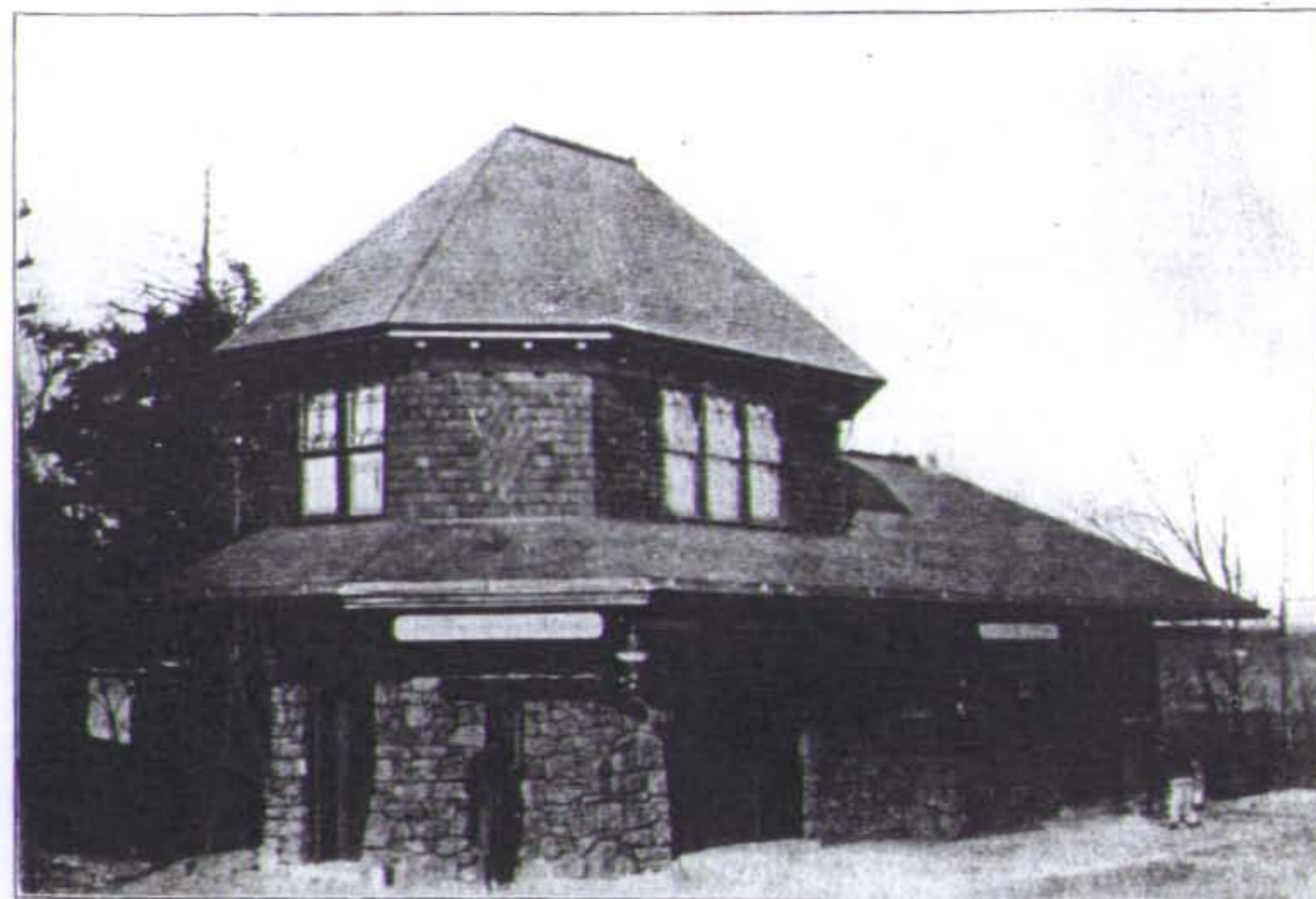
Photograph from Track Side of Station, as Completed.
