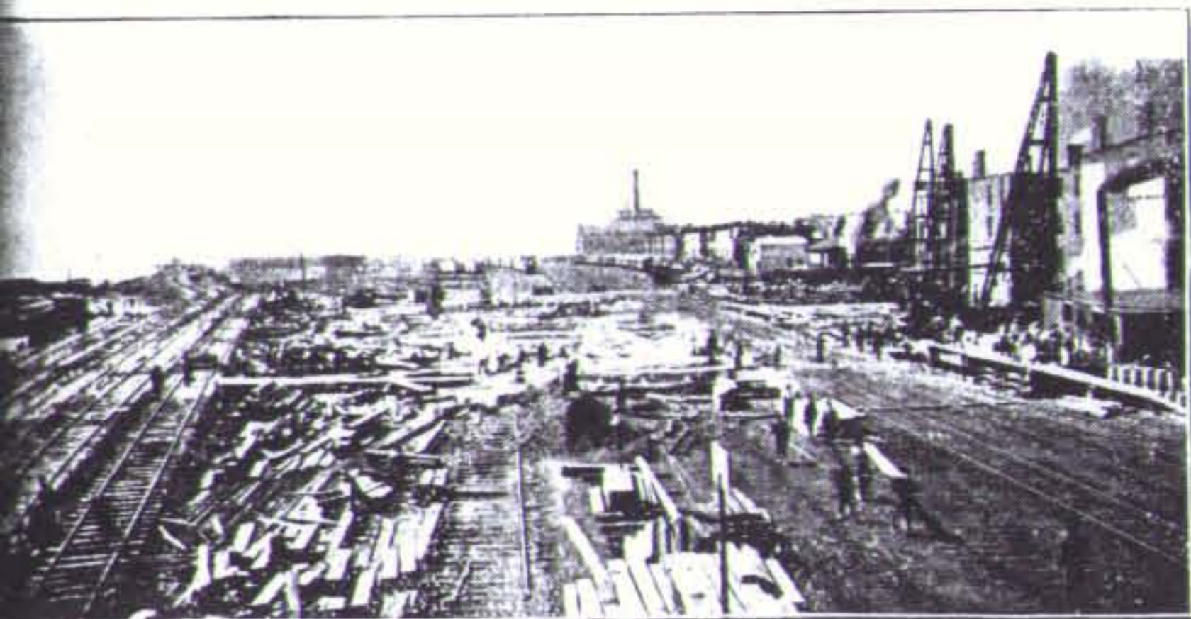
August 15, 1892. Completion of Pile Driving and Footings (Looking Toward the South).
