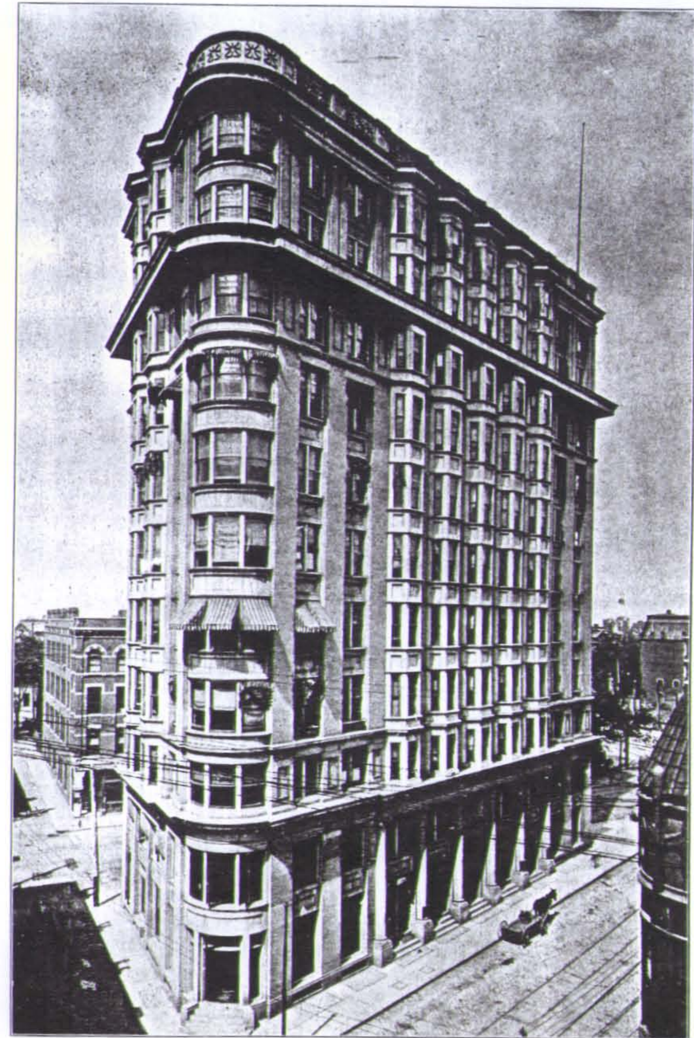
Flatiron, or Triangular Office Building. Erected 1896-97, Atlanta, Ga. Fire and Earthquake-proof Construction, 12 Stories in Height; Narrowest Point, 4\frac{1}{2} ft.; Sides about 145 ft., and Base about 60 ft. A Special Water Screen is Provided to Prevent Fire from Opposite Structures.
