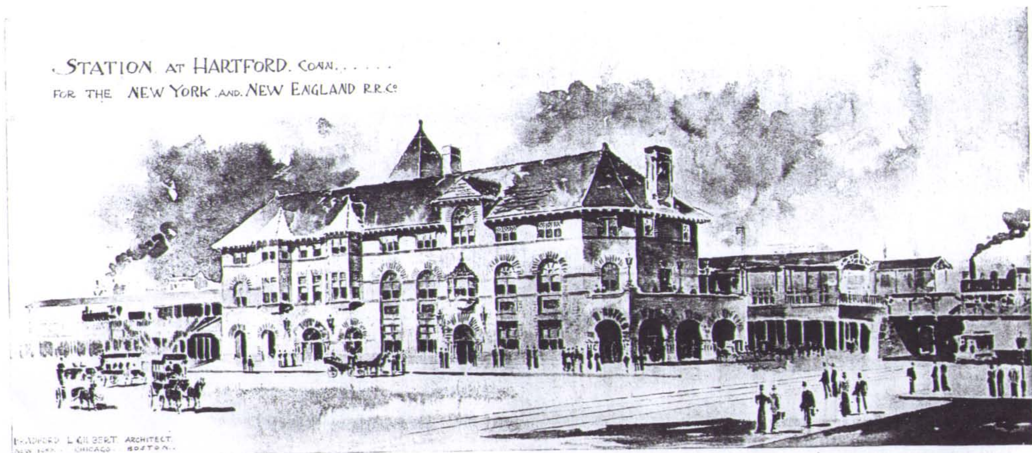
Proposed Construction: Of Buff Brick and Stone. Dimensions: 60 ft. x 220 feet. Three Stories in Height.
