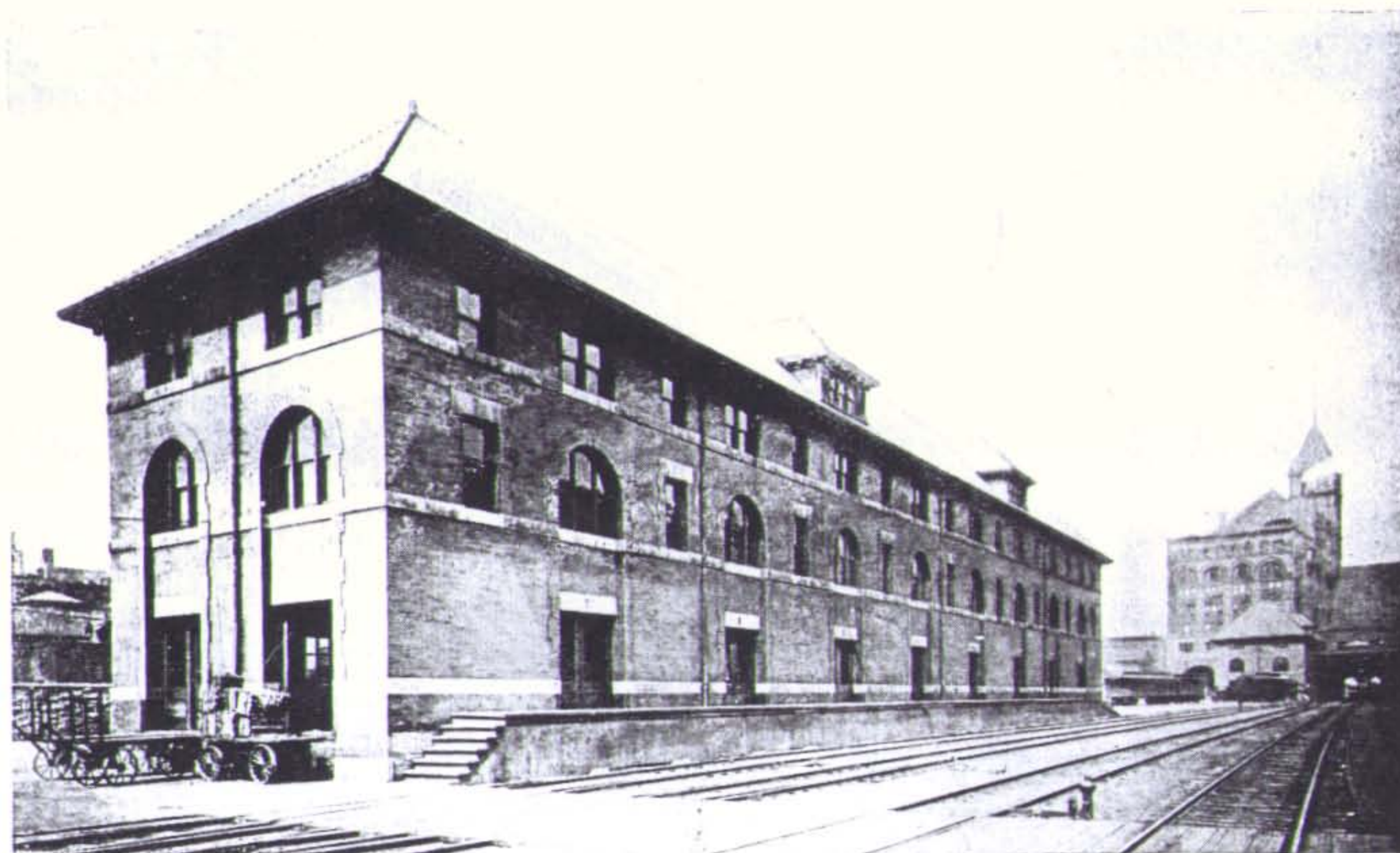
Construction: Of Brick and Stone. "Incoming" Building, 35 ft. x 210 ft. "Outgoing" Building, 48 ft. x 99 ft. Each Three Stories in Height with Baggage Elevators.
