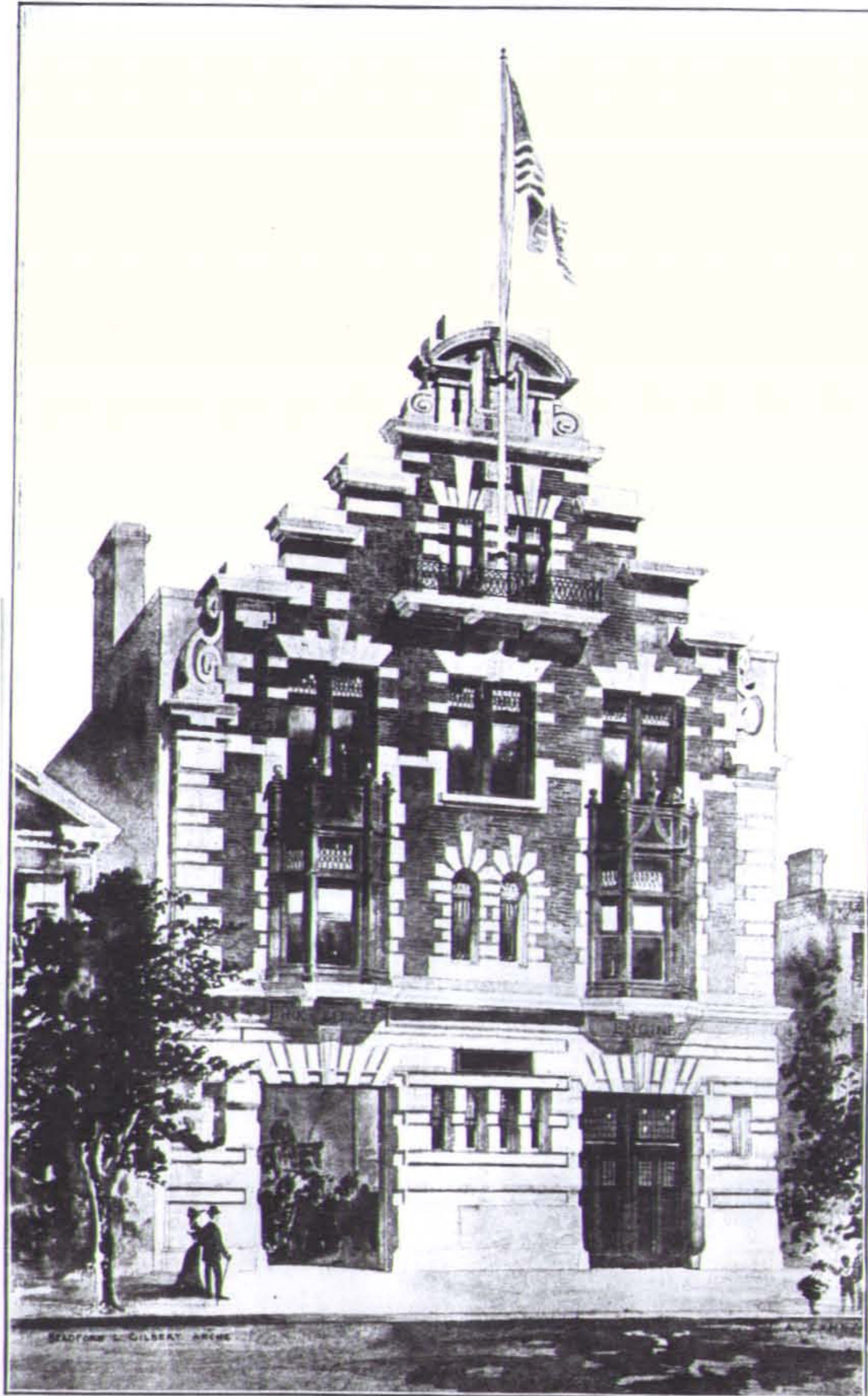
Double Apparatus House. Erected for New York City During 1903-04. Construction of Granite, Limestone, Cement and Brick.
