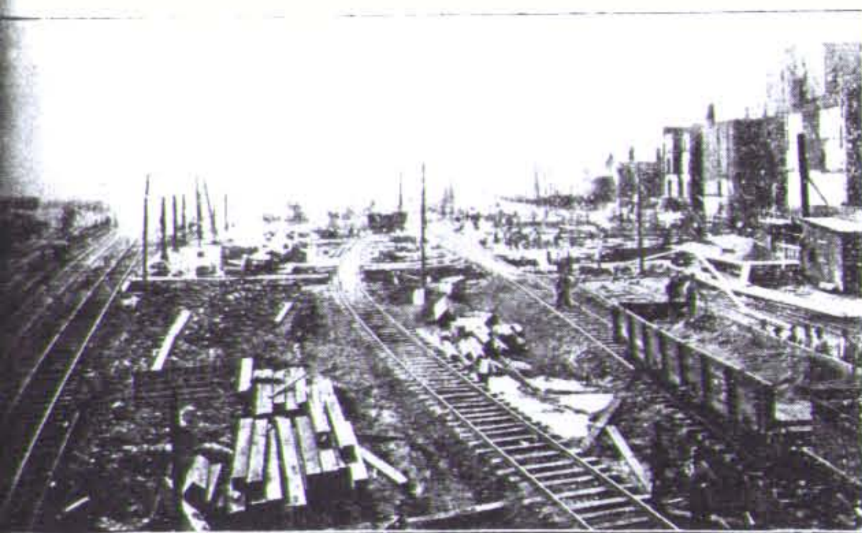
September 15, 1892. Erection of First Iron Columns Above Grade, and Basement Excavation Below.
