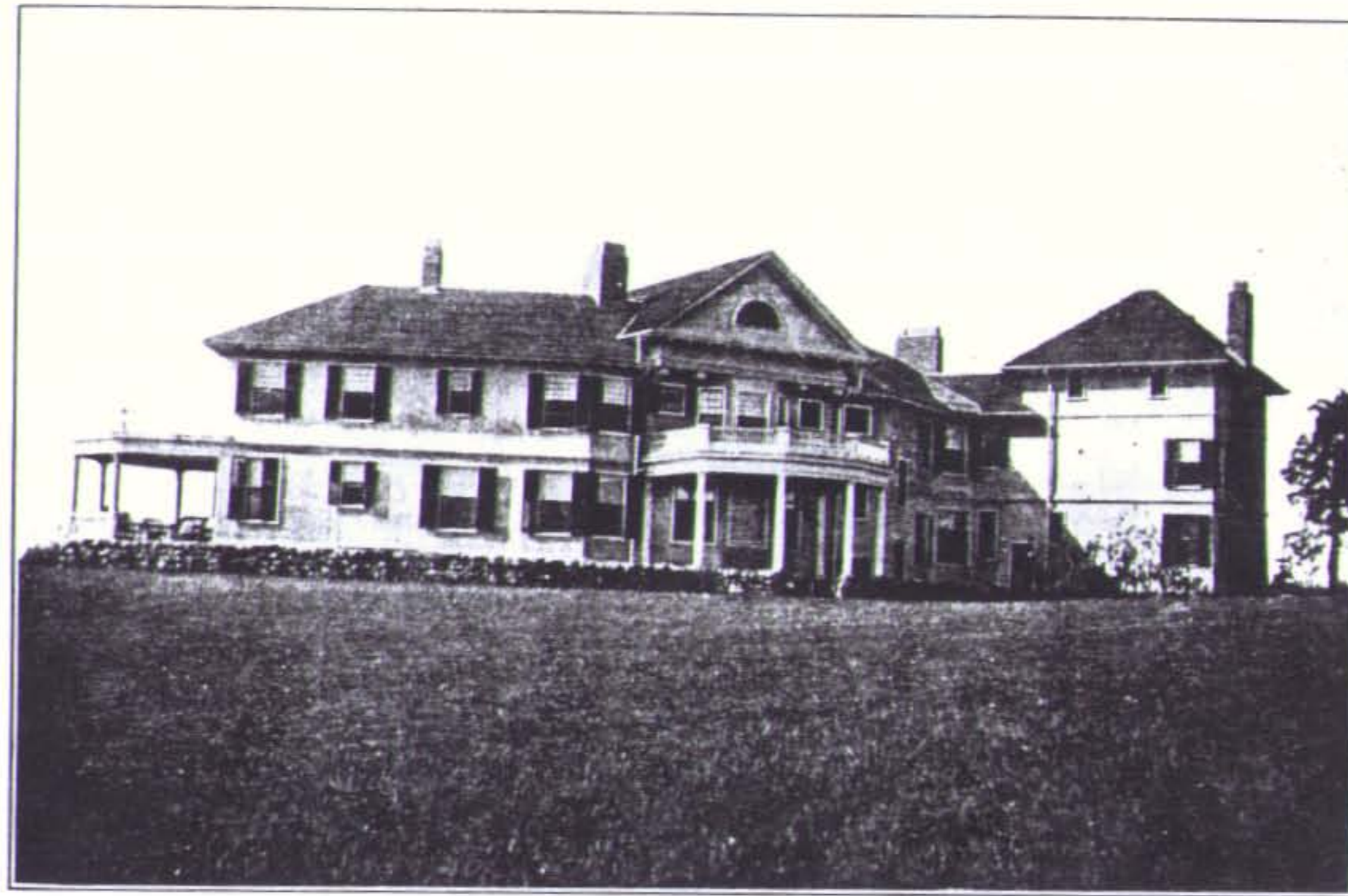
Home of Mr. W. H. Baldwin, Jr., from Photograph. Construction of Cement on Studs, without Sheathing; Roof, Gutters and Leaders of Cypress.
