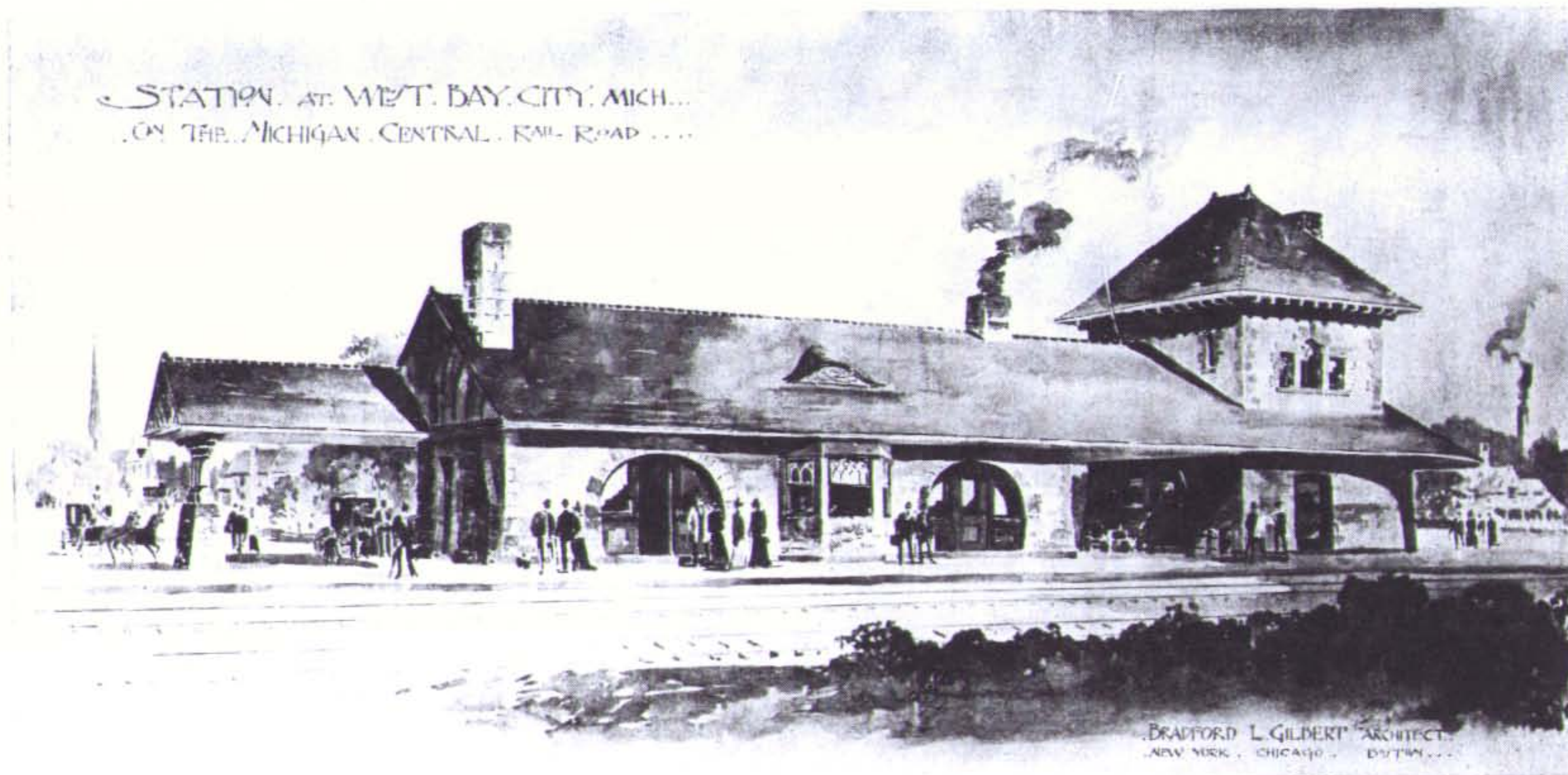
Construction: Of "Field Stone," with Dressed Stone Trimmings. Dimensions: 28 ft. x 120 ft. Exclusive of Port Cochere and Awnings.
