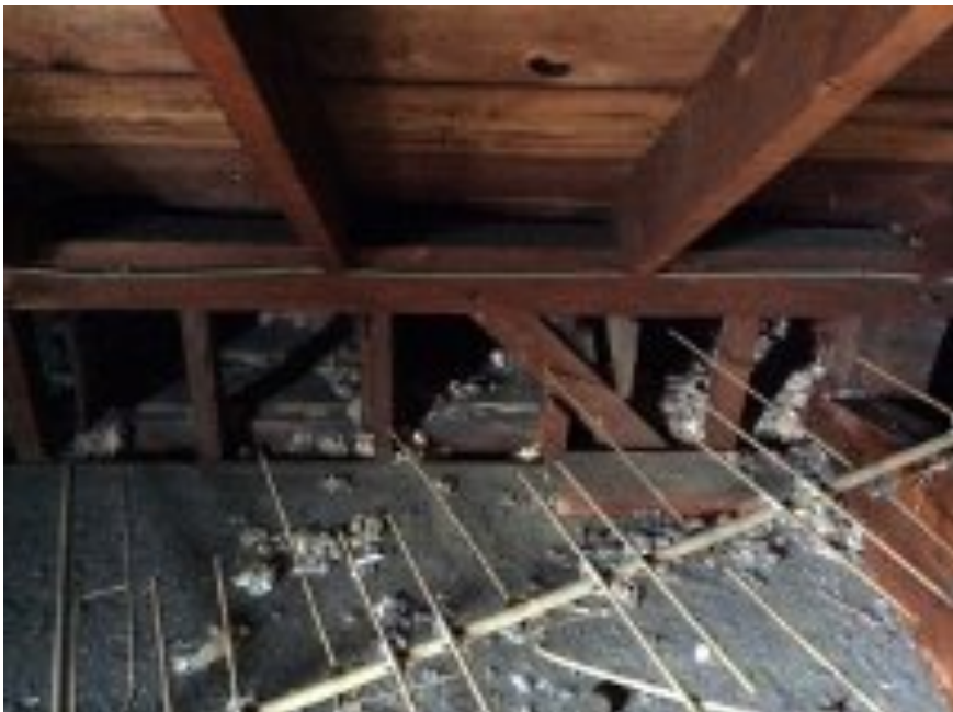
Photo 10. Fox-Seal General Store. Original block attic, north wall, eaves detail with cornice blocking.
