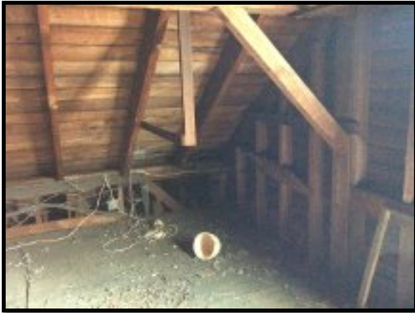
Photo 9. Fox-Seal General Store. Original block attic, SE corner, roof and wall framing, revealing original clapboard on west gable.
