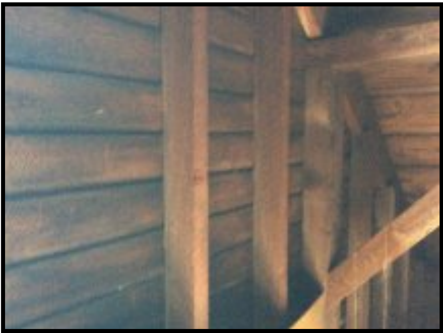
Photo 11. Fox-Seal General Store. Original block attic, west gable detail, revealing original clapboard siding, looking NW.
